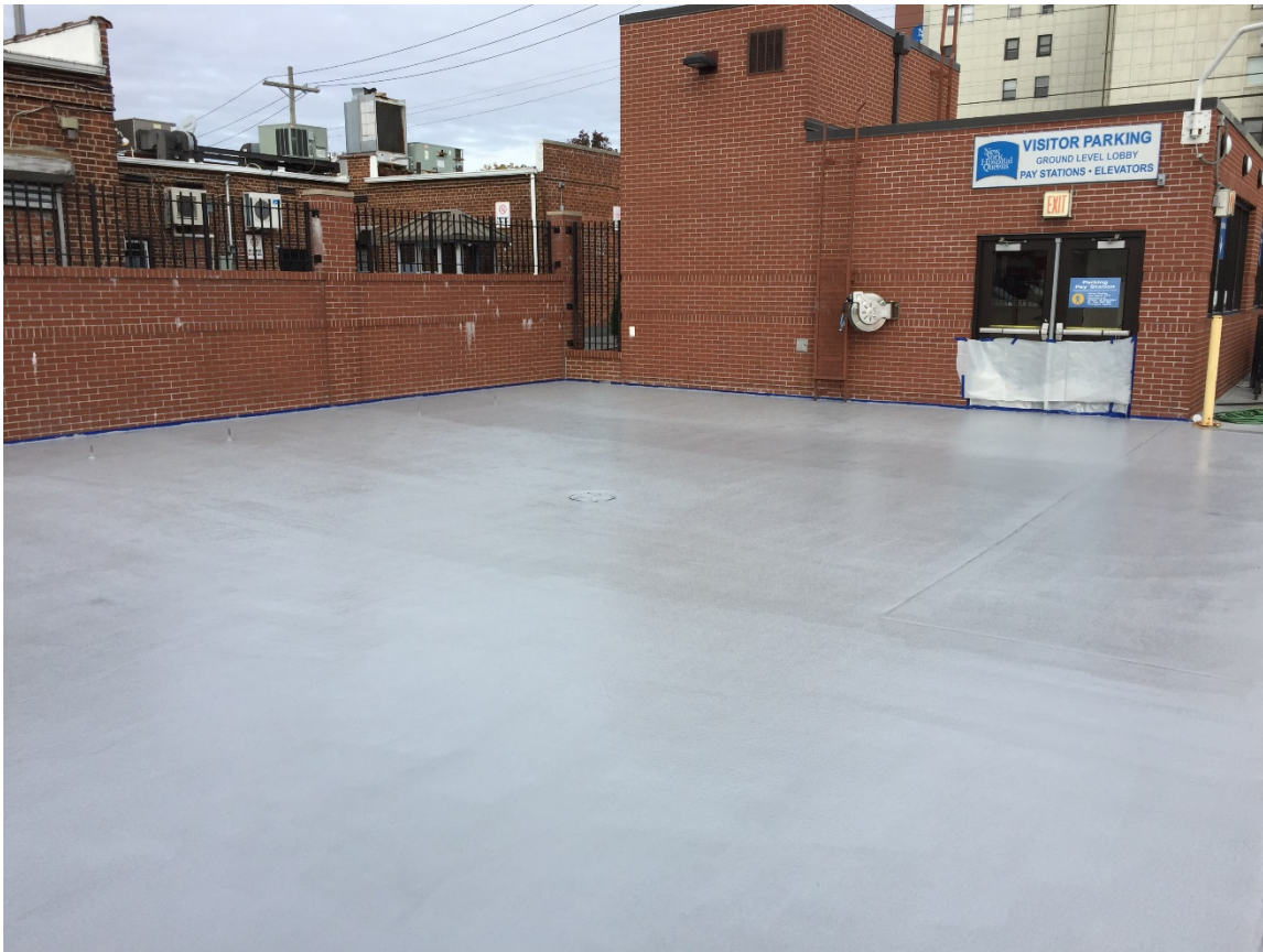
📍 Waterproofing overlay design at New York Presbyterian (Hospital) in Jamaica, New York
